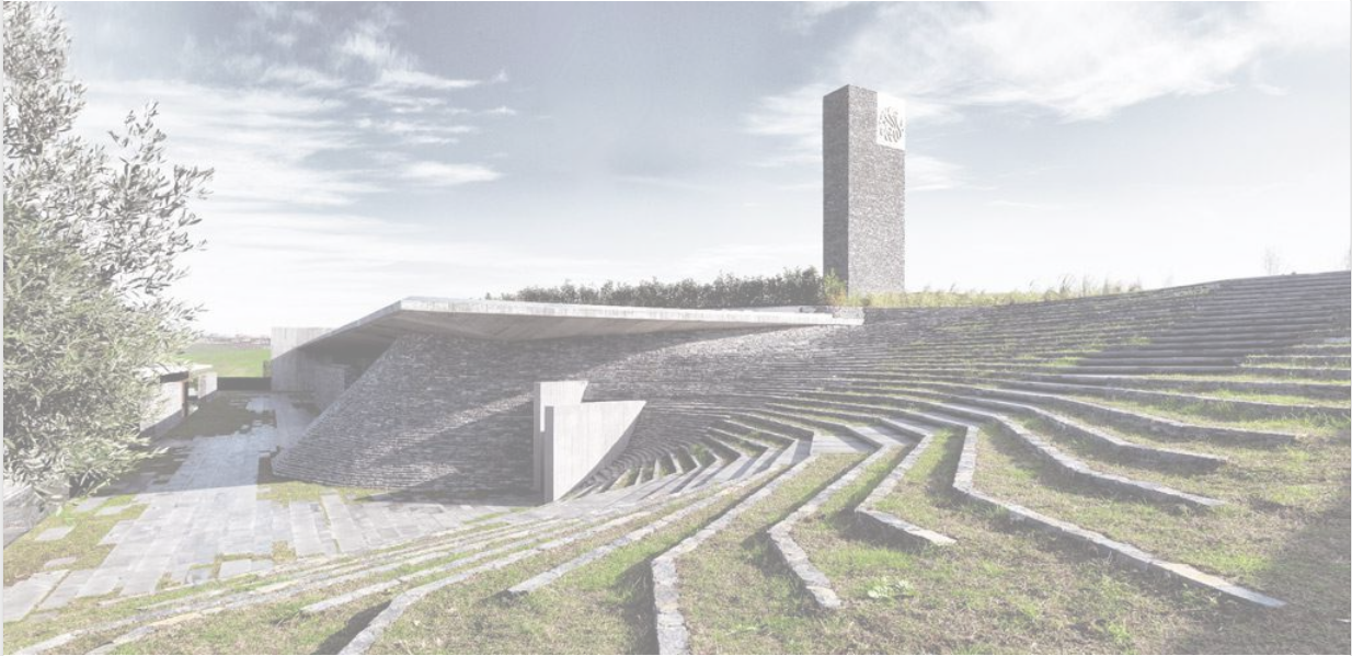
Emre Arolat's Sancaklar Mosque. Photo credit: Cemal Emden
